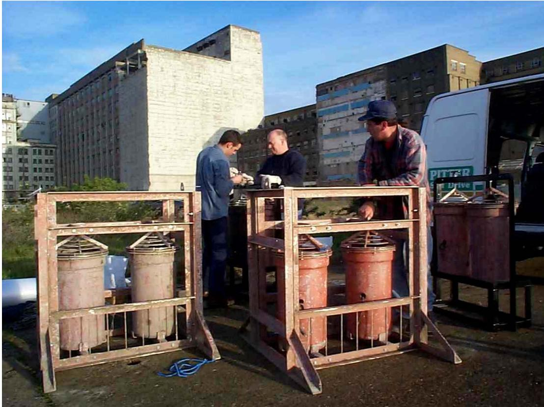
**Plate 3.13 Acoustic sound projectors being prepared for installation at Amer Power Station (The Netherlands) (courtesy Fish Guidance Systems Ltd)**
